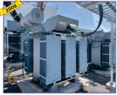
2100 kVA MF Pad Mounted Transformer
