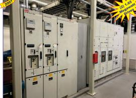
ABB Frequency Drive System with Related Switch Gea
